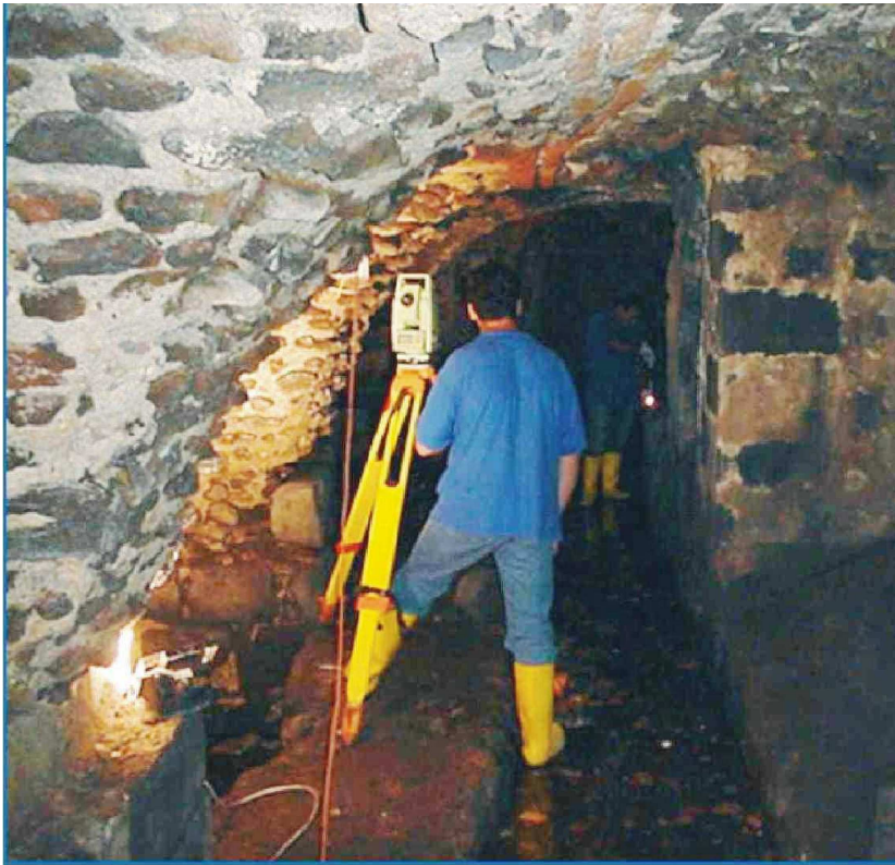
Fig. 2a. Structure of the arcs of the Thermae is in terra cotta bricks and the vault in blocks of lava stone.
